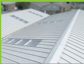
ANY TYPE OF OLD & NEW SHEET ROOFING & RCC ROOFS
